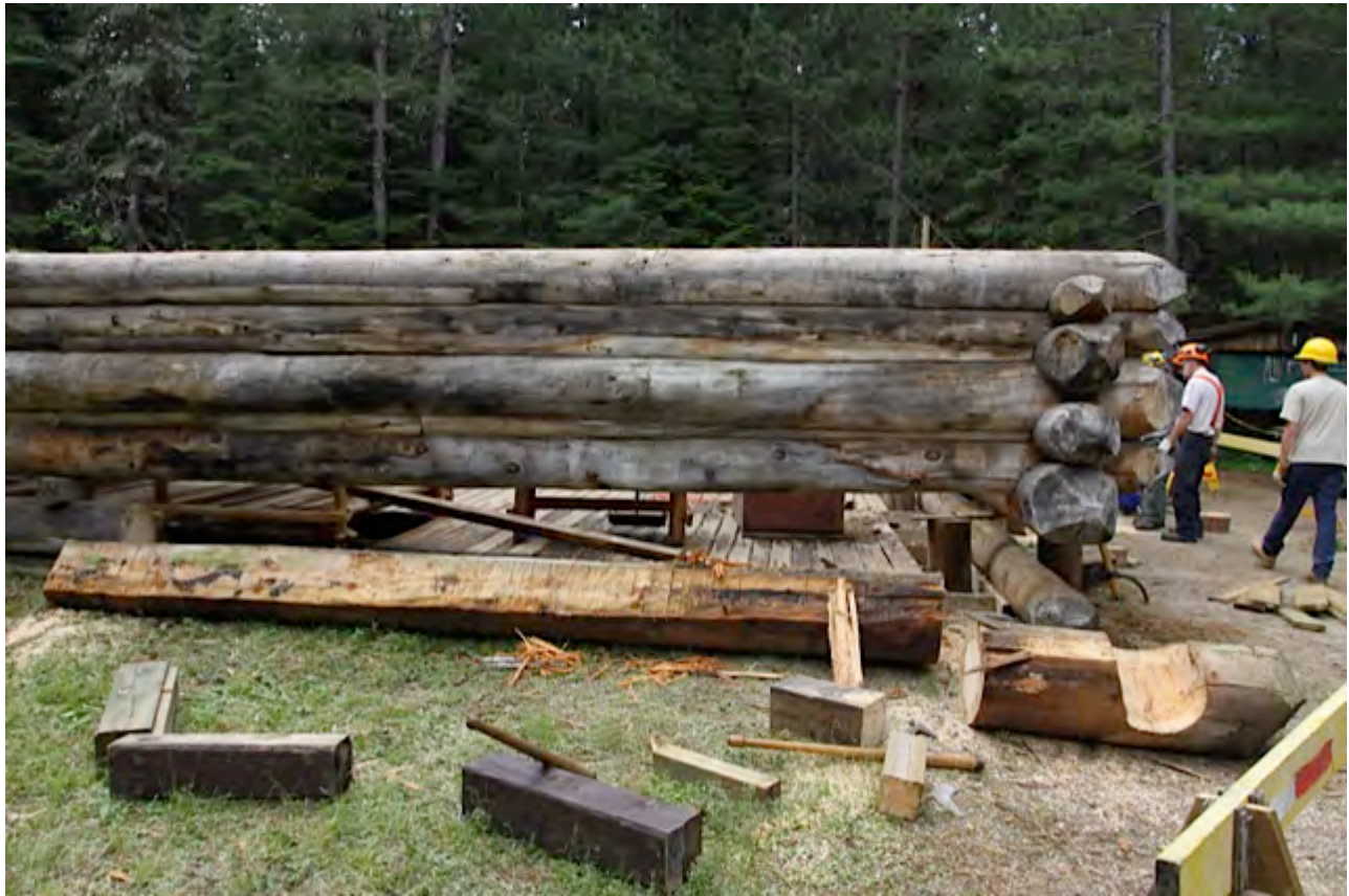
Figure 2: Repairs to the Algonquin Park Logging Museum Camboose Camp
